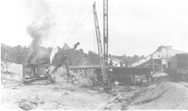
Author's photo, Bucyrus 225-B being erected
